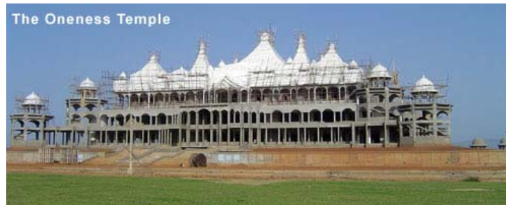
The oneness Temple while under construction
